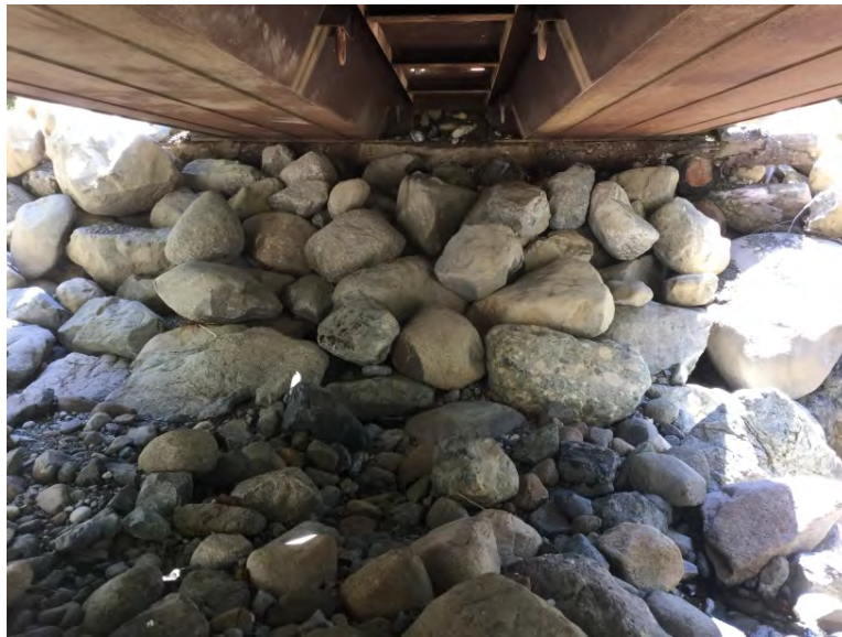
Left Bank Abutment when facing downstream
